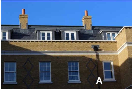
A - A good quality response to dormers – proportionate, set back from the eaves, aligning with fenestration of the façade and reflecting historic vernacular
